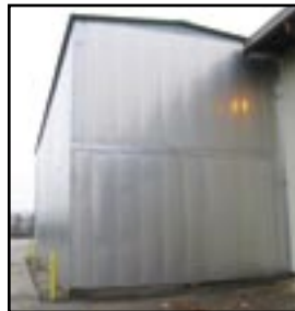
Gas Fired Ovens
