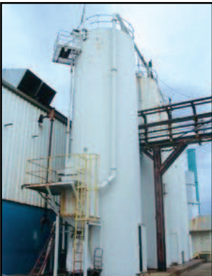
View of Silos
