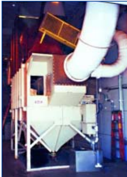
AAF Rotoclone Wet Type Dust Collector, Mdl. #B
