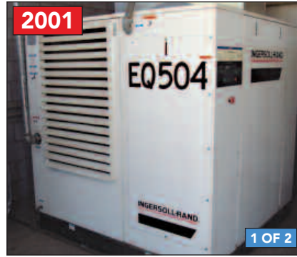
INGERSOLL-RAND 50-HP AIR COMPRESSOR
