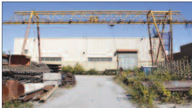
10 TON HEEDE / P&H OUTDOOR DOUBLE LEG PORTAL CRANE
