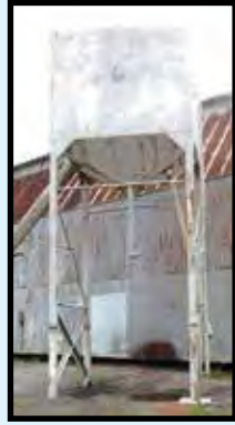
SANDBLAST GRIT TOWER
