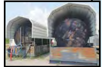
OILY WATER STORAGE TANKS
