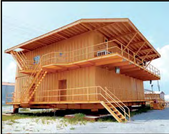
PORTABLE OFFICE BUILDING
