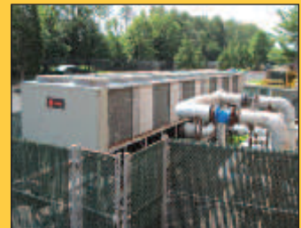
TRANE AIR COOLED PROCESS CHILLER
