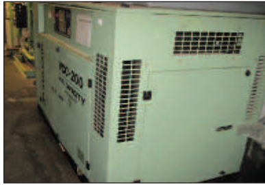
SULLAIR 100-HP ROTARY SCREW AIR COMPRESSOR
