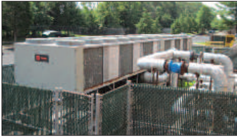
TRANE RTAA400, 400-TON AIR COOLED PROCESS CHILLER
