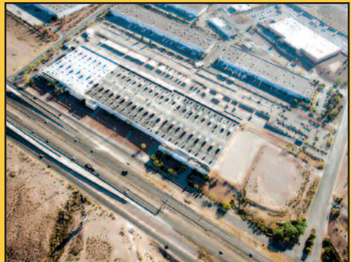
AERIAL VIEW OF FACILITY
