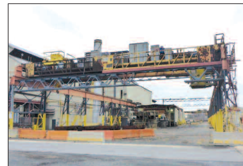
ALLIANCE 20 TON OVERHEAD BRIDGE CRANE
