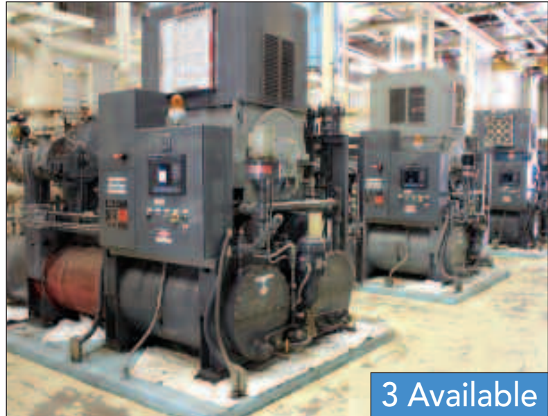
ATLAS COPCO HL-7 CENTRIFUGAL AIR COMPRESSORS, 1,250-HP
