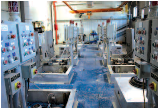
SPINNING TOWER AREA
