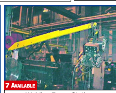
7 AVAILABLE Welding Boom Stations
